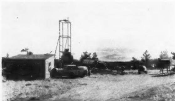
BLUE JAY mine where the vertical shaft is now being deepened to new contact. Pikes Peak shows 40 miles east.
